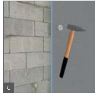
C Place wedi Tools metal dowels in the holes and hammer in after the mortar has fully dried.
