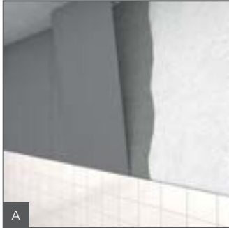
Attach the building boards across the full surface with tile adhesive.
